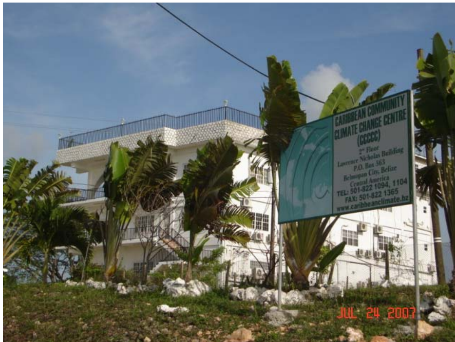
Figure 1 Building housing the offices of the Climate Change Centre
