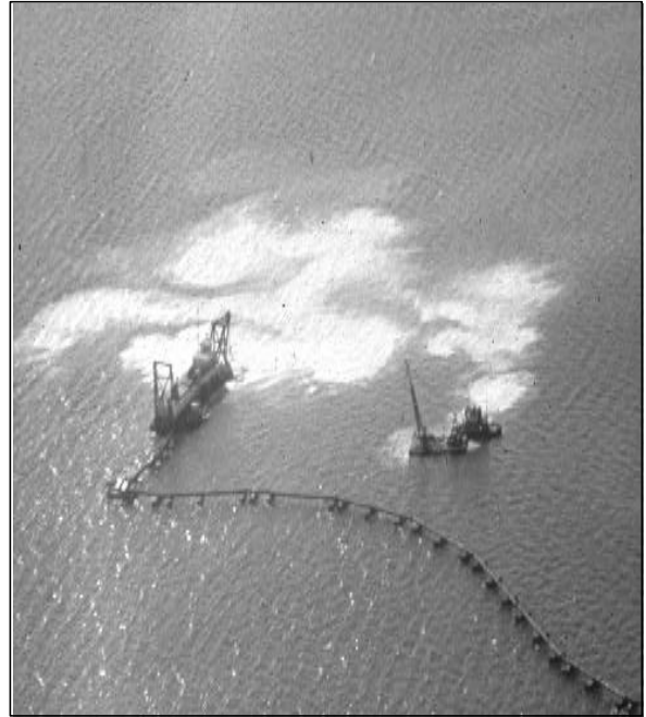
Figure 3-8. Sediment plume associated with dredging in North Sound, Grand Cayman. (Photo from DOE collection).
